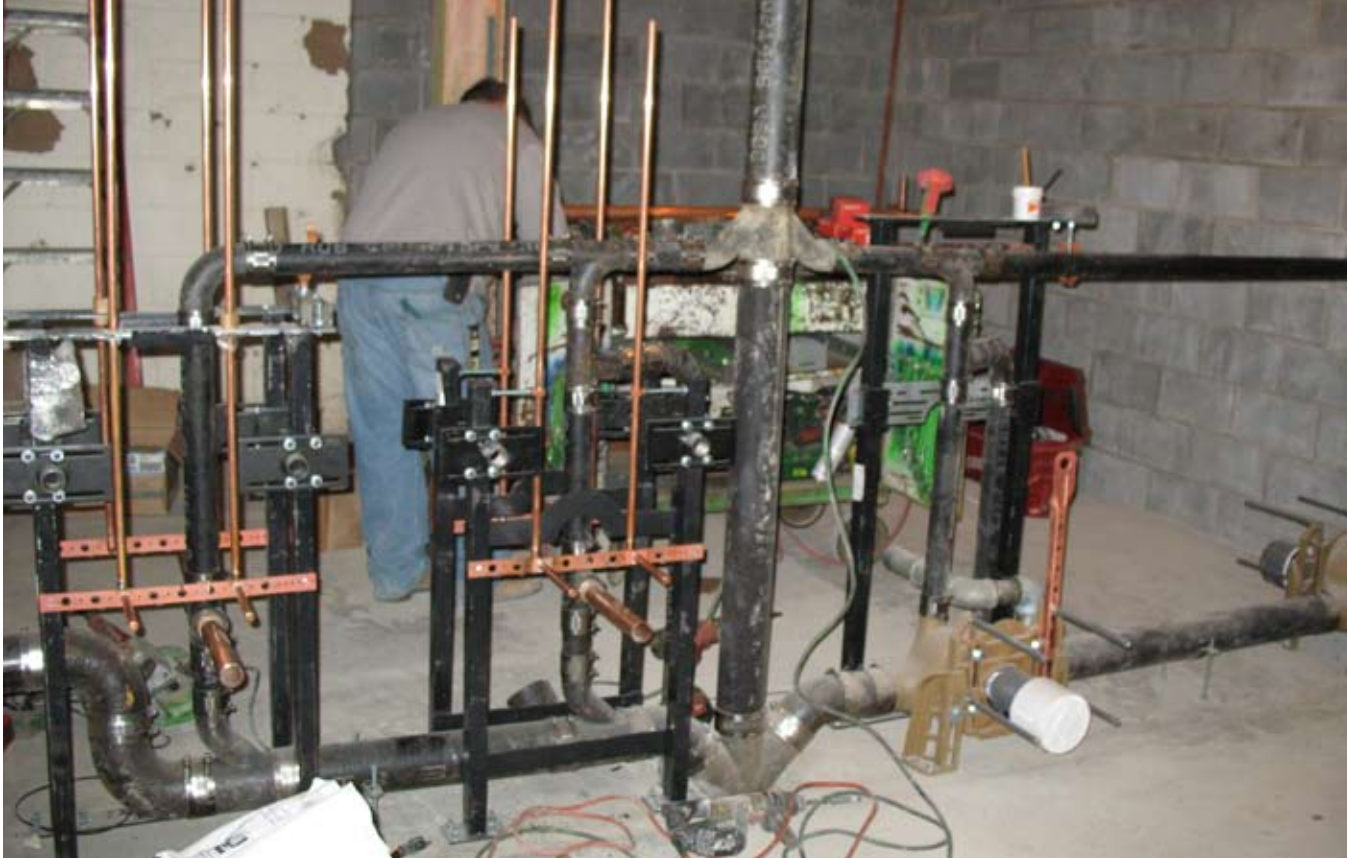
Jay R. Smith Mfg. Co.® Labor Saver Fixture and Water Closet Supports used by Evans Mechanical.
